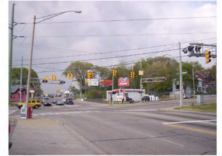
4. Intersection of Plainfield and Leonard - Looking North
