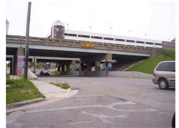
24. Lafayette at I-196 Overpass - Looking South
