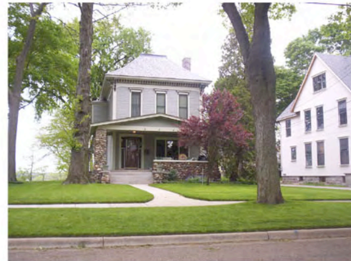
15. Single-Family Residence on Fairview - Looking West
