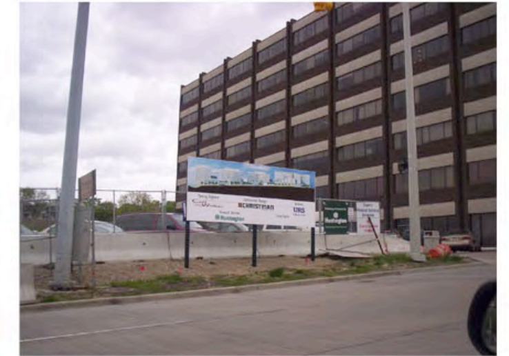
8. Spectrum Construction Site on Michigan - Looking North
