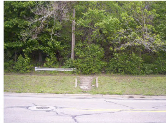
6. Newberry Stairs - Looking East
