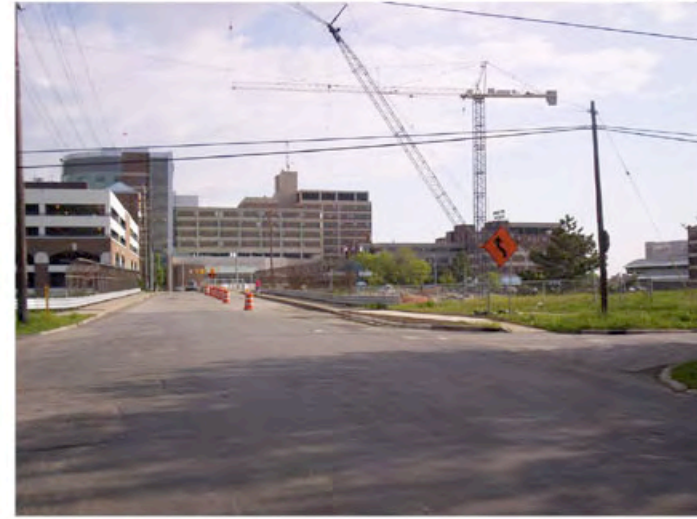
2. Coit Street Bridge over I-196 - Looking South
