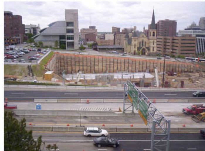
14. Spectrum Construction Site and I-196 - Looking South from Hastings Street
